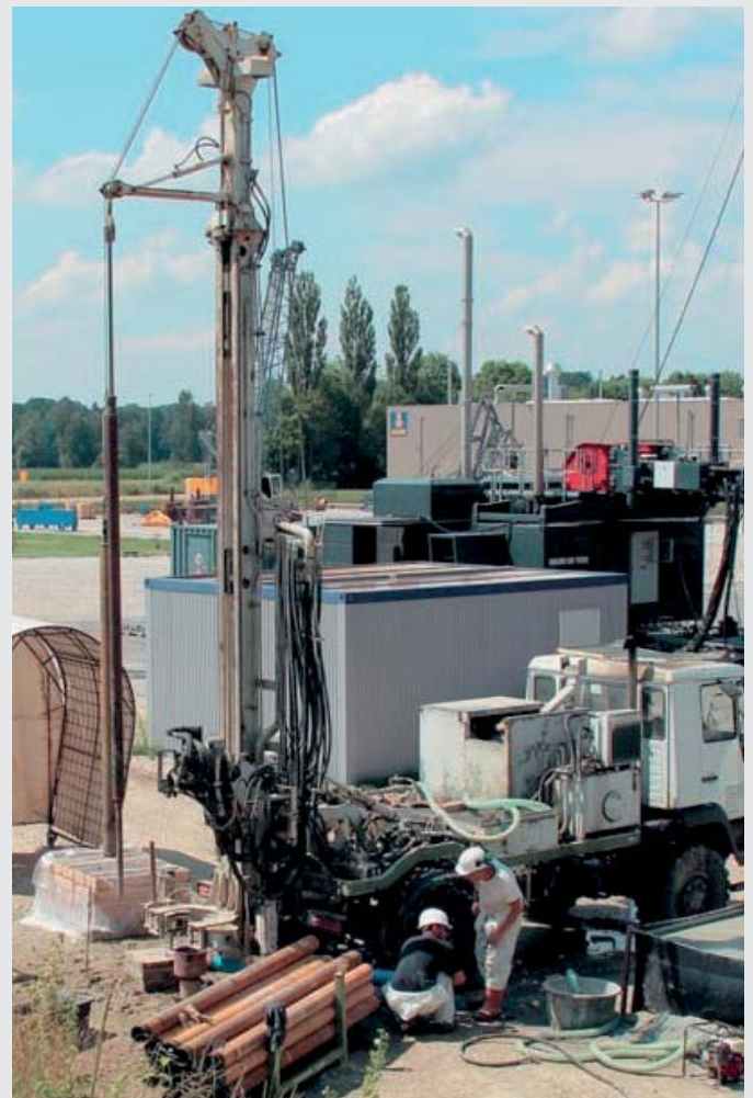
Vertical core drilling with a drill rig for exploratory boreholes
