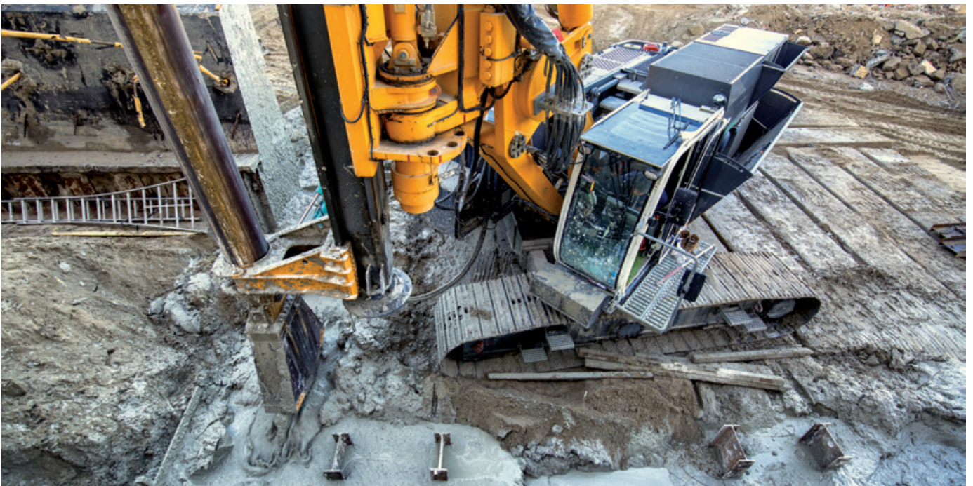
Corner formation retaining wall
