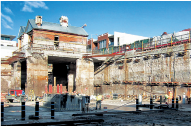
Retaining wall and underpinning for a heritage building
