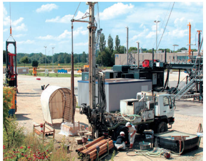
Drilling "vertical" core holes
