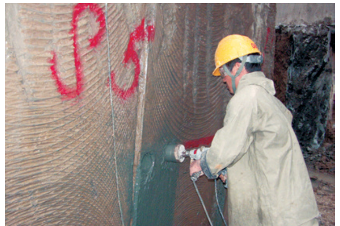
Horizontal core sampling with a hand-held drill
