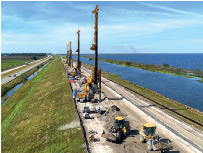
Cut-off wall for dyke rehabilitation
